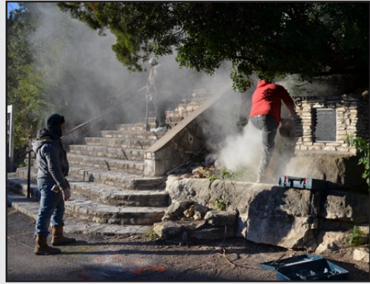
As soon as the ceremony was over, experts from Beall Memorial Art started work on constructing the monument.
